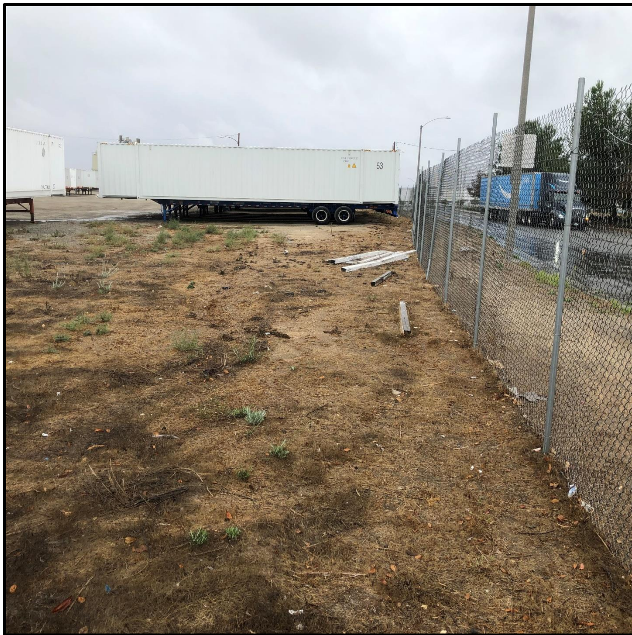
Figure 4.1-5 WEST SIDE OF THE PERIMETER, SOUTH HALF; VIEW TO THE NORTH
