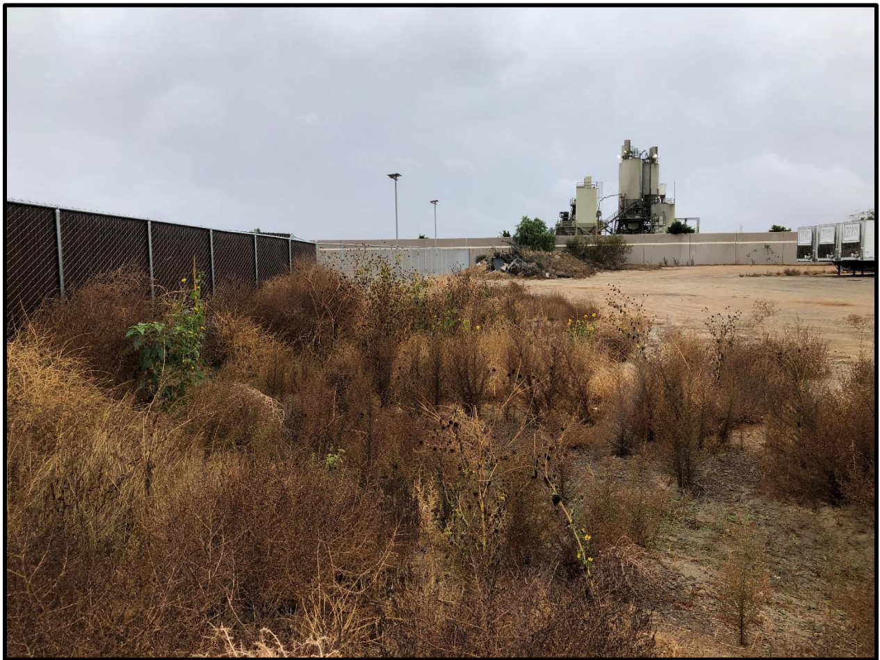
Figure 4.1-3 EAST SIDE OF THE PERIMETER, SOUTH HALF; VIEW TO THE SOUTH
