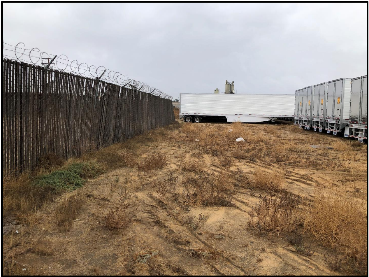
Figure 4.1-2 EAST SIDE OF PERIMETER, NORTH HALF; VIEW TO THE SOUTH
