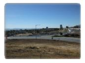
west side of Moreno Beach Drive, the contractor has cleared the area for the new eastbound off-ramp. The goal of the project is to realign the eastbound on- and off-ramps to a "diamond" configuration and complete the connection of Eucalyptus Avenue to Moreno Beach Drive, thereby providing better access to the area. Due to several rainy days, if the time is not recovered, construction will extend to mid-September 2013.
