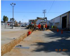
Technology Services and the Public Works Maintenance and Operations crews worked together at the City Yard to excavate a 140-foot trench for installing underground conduit that will soon carry fiber optic cable. The 140-foot conduit
