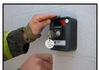
A Knox Box is basically a locked key box. The purpose of a Knox Box is to provide the Fire Department with rapid, non-destructive access to the property and building during emergency situations. Property owners can put all necessary keys, pass cards, and other relevant items in a Knox Box to ensure efficient, effective after-hour entry should emergencies occur. If you open a new business or multi-family dwelling such as an apartment building or
