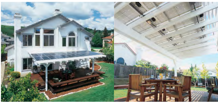
A solar porch or patio roof is an attractive option and avoids placement of system components over roofing.
