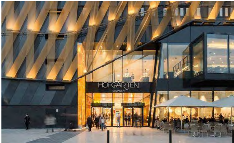
Example of an activated mall entryway.
