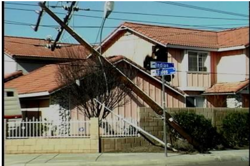
Downed power pole causes power outage in Moreno Valley due to high winds January 2003 (source MVTV-3)
