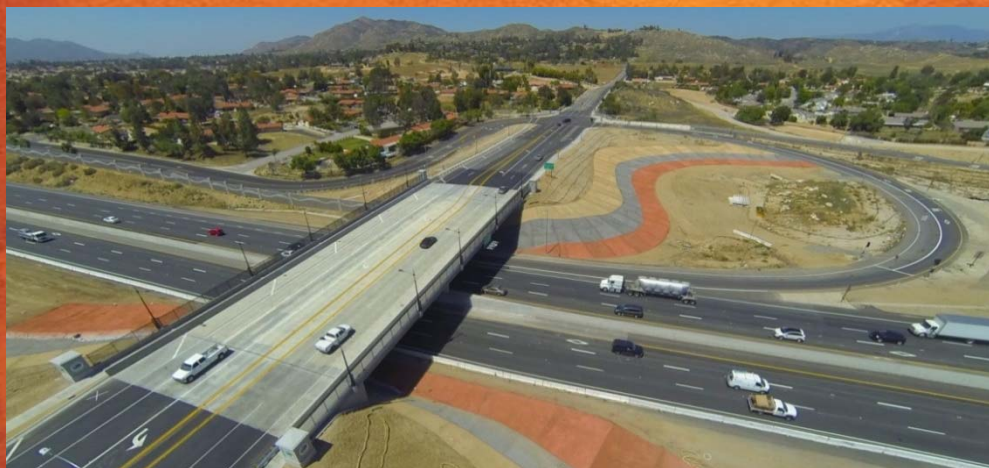
SR-60 / Nason Street Overcrossing Bridge
